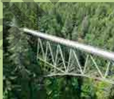
High Steel Bridge, a truss arch bridge above Skokomish River in Washington, USA
