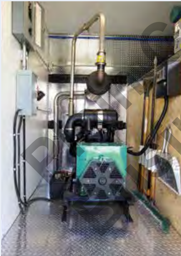
↑ A generator sits inside one of the partitioned areas of the insulated trailer. Image Source: Leroy Martin
